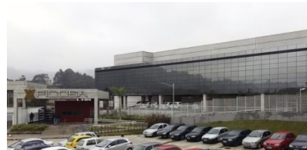
Brazil New Plant
